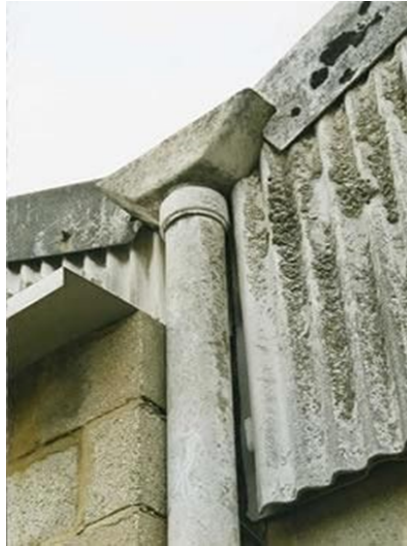
Asbestos cement downpipe, hopper and profile sheet
