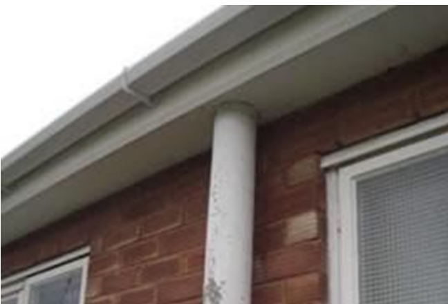
Asbestos cement drainage pipe (downpipe)
